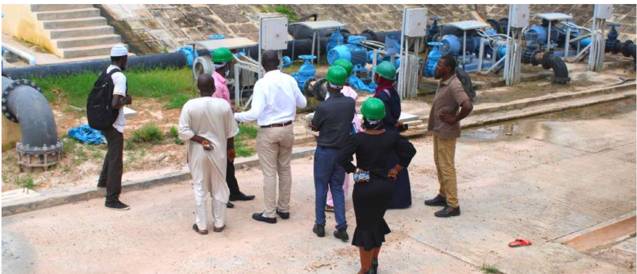
A visit to Sukuta Treatment Plant
