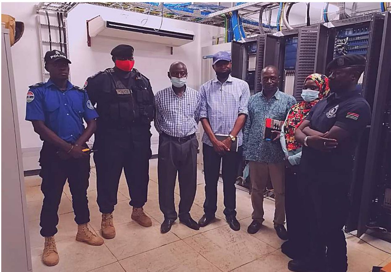
Monitoring Team at the Comium Server Room
