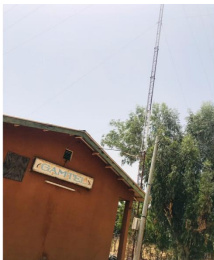
GAMTEL exchange station at Illiasa, NBR
