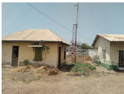
GAMTEL exchange station at Kuntaur, CRR
