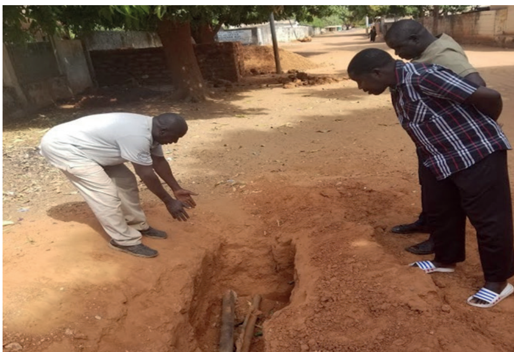
Figure 52: Inspection of the pipe network before the replacement
