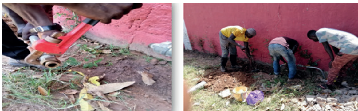
Figure 51: NAWEC Plumbers Changing Non-return valves
