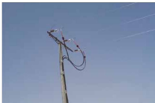
Figure 26: Underground cables from Senegal linking to the NAWEC grid at Amdalai to supply the North Bank
