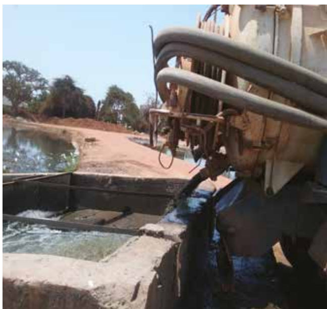
Figure 44: Discharge in progress at the Second pond skipping one of the key steps of pre-treatment.
