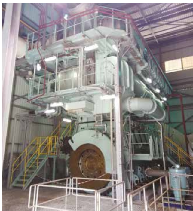
Figure 30: Brand new 11MW engine commissioned in Kotu
