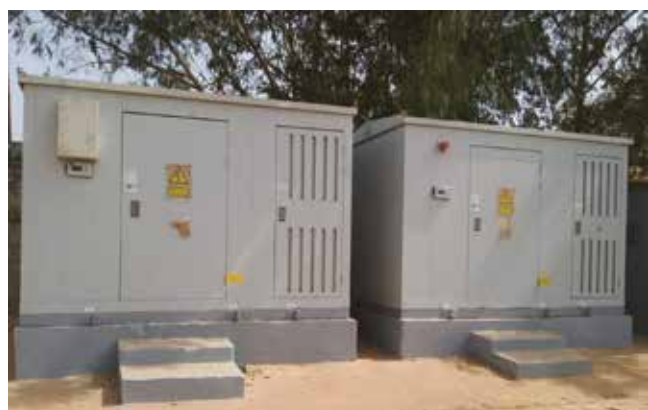
Figure 25: switchgear and metering points on the interconnection from Senegal at Keer Ayub/ Farrafeni crossing.
