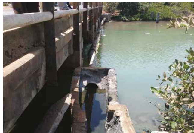
Figure 45: Exposed manhole along the kotu Silo Bridge with the sewage pipe under the bridge
