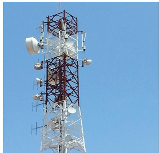
Figure 18: BTS cell site with antennas
