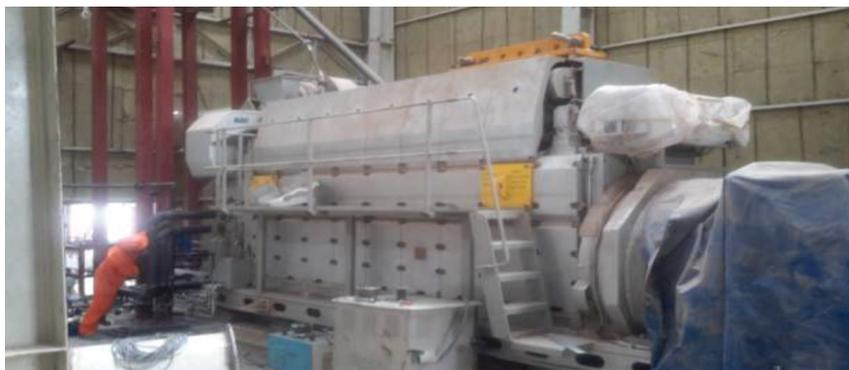
Figure 22: The new MAN 2.3MW engine HFO engine at Farafenni being installed
