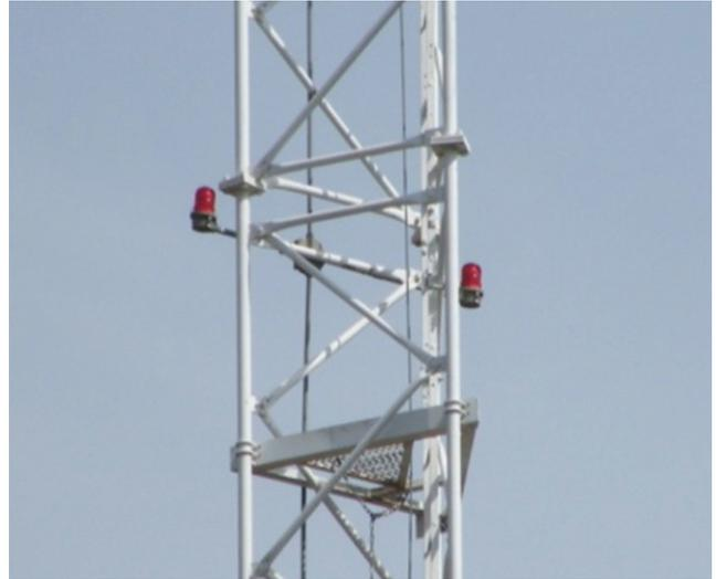
Figure 20: Mast showing aviation safety red lights (25m and above)
