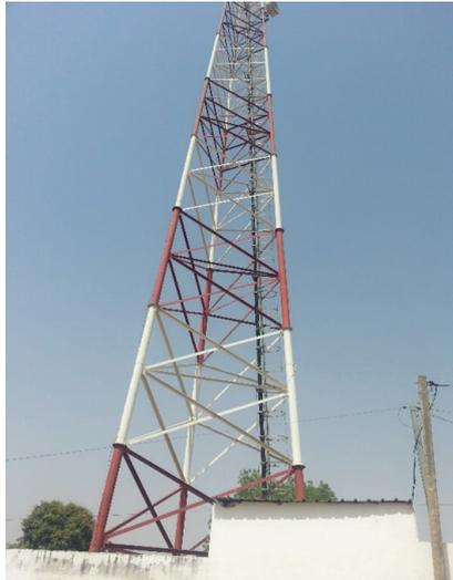
Figure 19: Tower showing alternate red / white aviation safety paint
