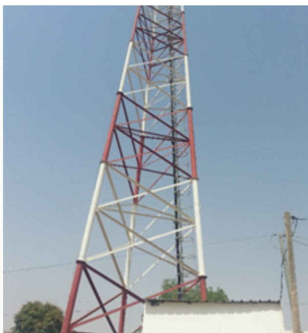
Figure 24: Tower showing alternate red / white aviation safety paint
