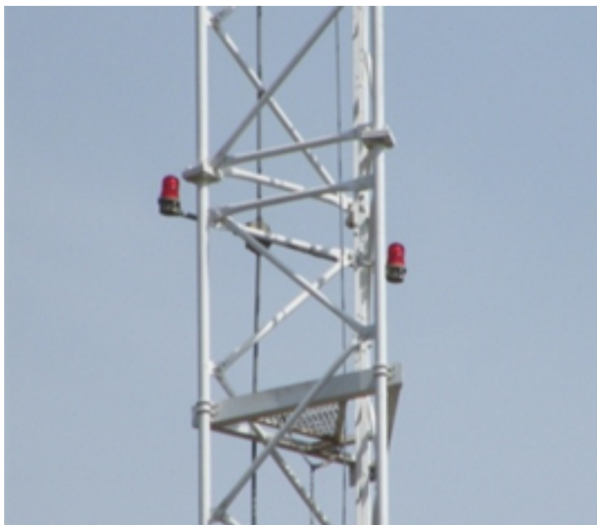
Figure 25: Mast showing aviation safety red lights (25m and above)
